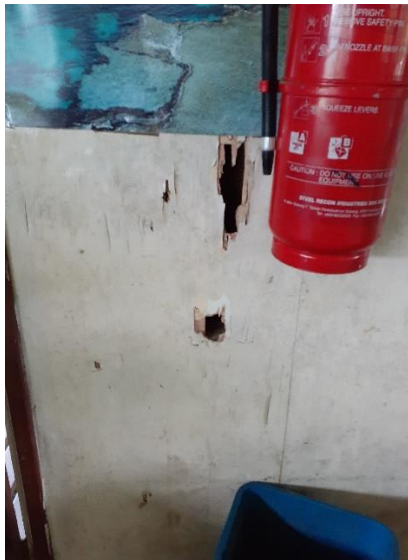
Prep classroom wall damage
